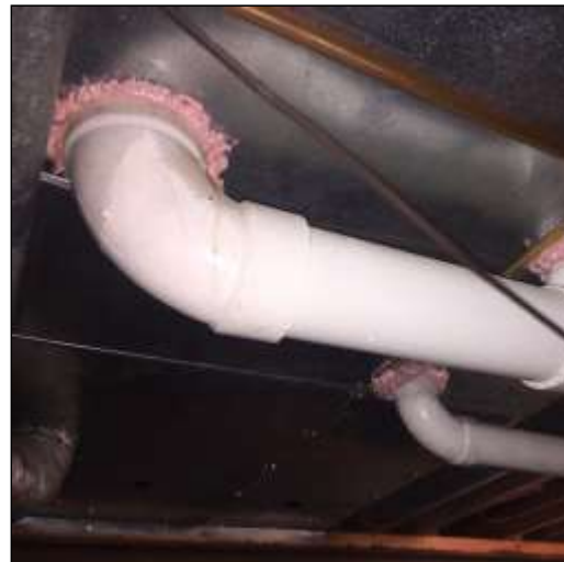
Figure 2 Foam Used To Seal Large Holes
