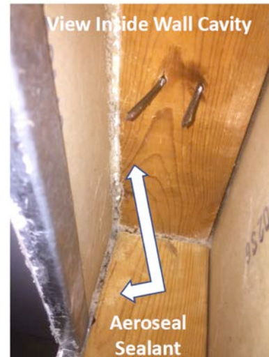
The aerosol sealant locates and seals leaks throughout the air distribution system.
